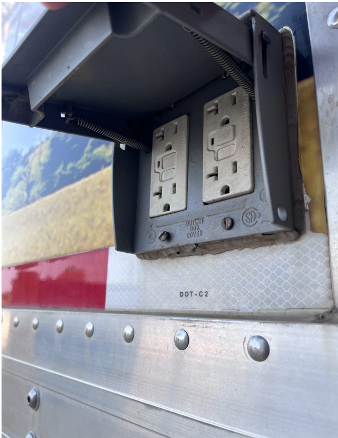
Exterior weather-protected duplex receptacles / utility outlet panel on all for exterior corners.
