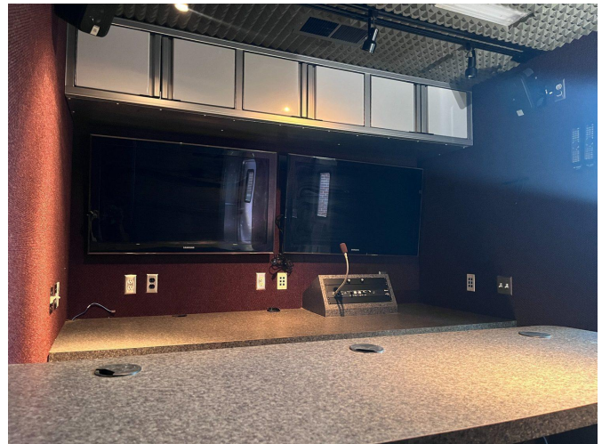
Current production desk / monitor-wall area after removal of some legacy electronics.
