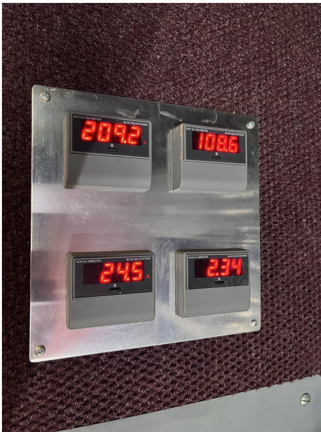
Blue Sea Systems digital AC voltmeter/ammeter panel; energized readings are visible in the photo.
